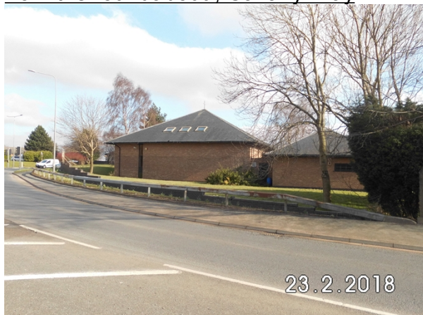
Church buildings (St Teresa's) seen from the roundabout , Cavalry Way
